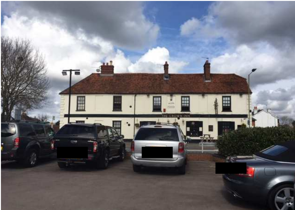
View from application site to north towards Church Street
