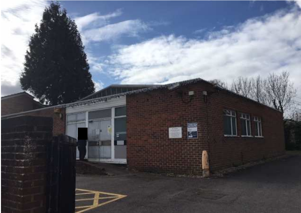
View of adjacent building to south of site from Station Road
