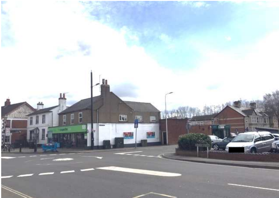
Buildings to east of site from Church Street towards Station Road and High Street
